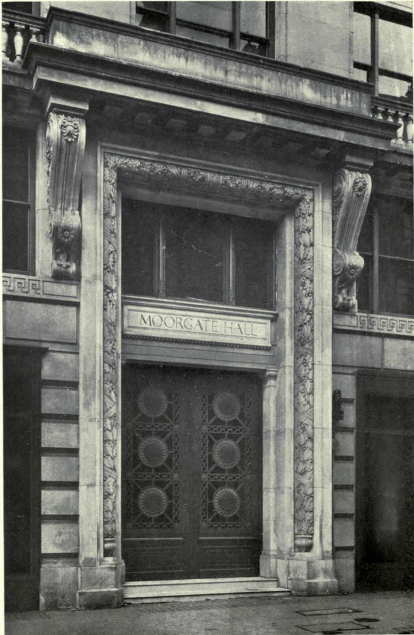
MOORGATE HALL, MAIN ENTRANCE : DETAIL.
